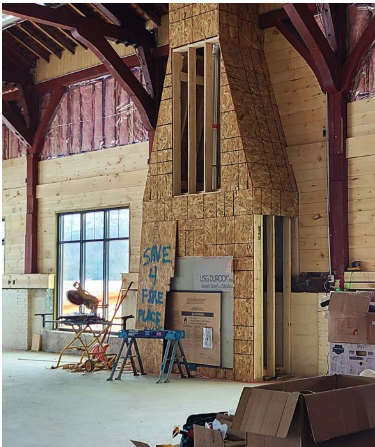
Above: The grand fire place framed up during construction.
